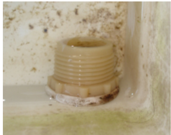
Photo 12 – Tap fixed using the reduction
